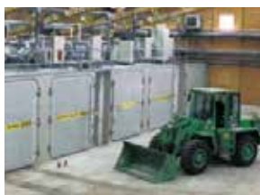
Intensive composting in Herhof composting boxes
